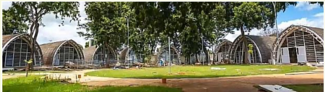
SESC Poconé school project: aspects of the circular square with surrounding buildings, giving children the opportunity to familiarize themselves with the design of the village.
